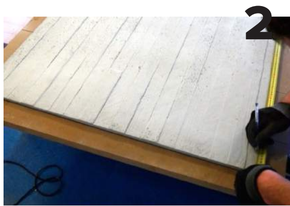
— COPY YOUR MEASUREMENTS ON THE PANBETON®
