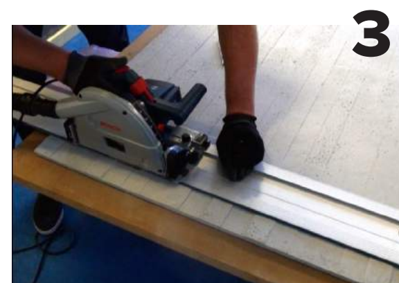
START CUTTING WITH A PLUNGE-CUT SAW
