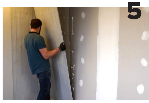
— INSTALL THE PANBETON® BY STARTING FROM BOTTOM TO TOP
