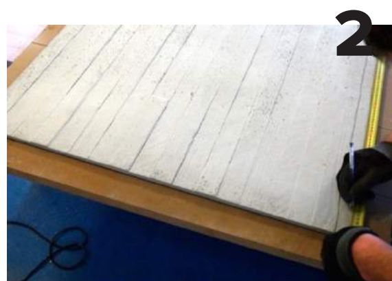
COPY YOUR MEASUREMENTS ON THE PANBETON®
