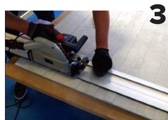
START CUTTING WITH A PLUNGE-CUT SAW
