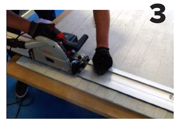
— START CUTTING WITH A PLUNGE-CUT SAW
