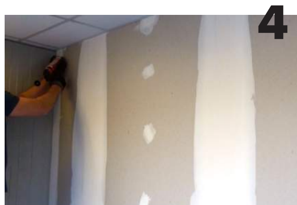
— APPLY GLUE ON THE WALL
