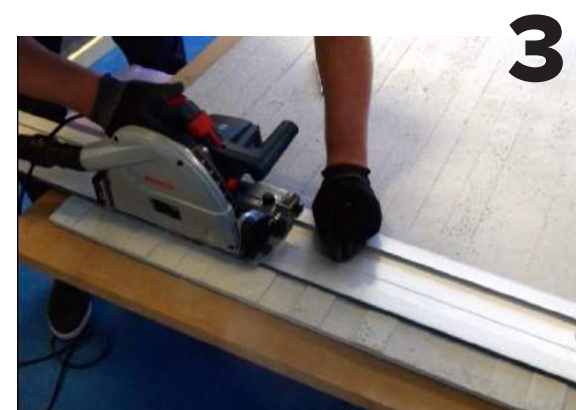
— START CUTTING WITH A PLUNGE-CUT SAW
