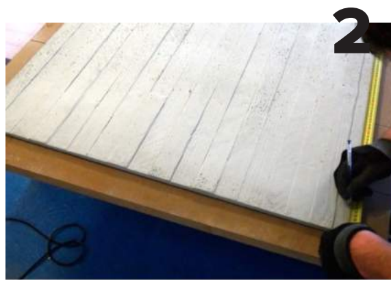
— COPY YOUR MEASUREMENTS ON THE PANBETON®
